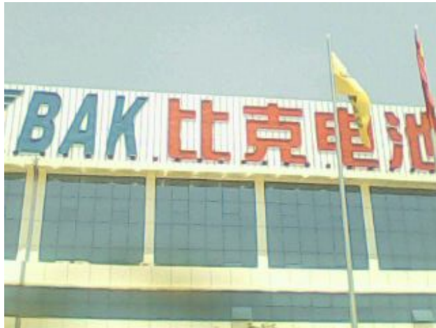
The Shenzhen Bak Battery building
